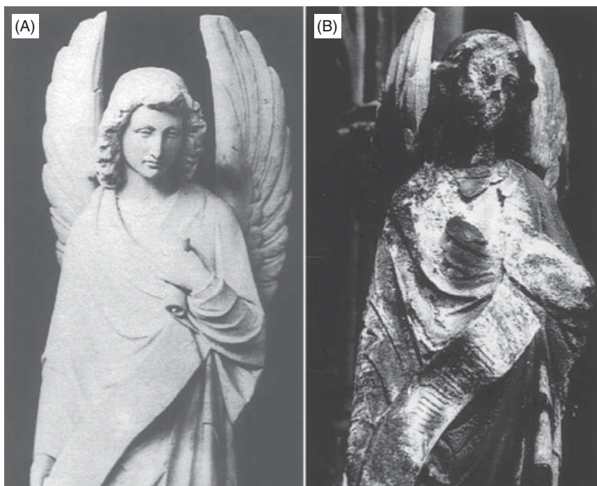
Figure 6.1 Effects of pollution caused deterioration on the statue of an angel at the cathedral of Cologne, Germany: (a) picture taken in 1880; (b) the same statue in 1993. (From Warscheid and Braams, 2000.)
